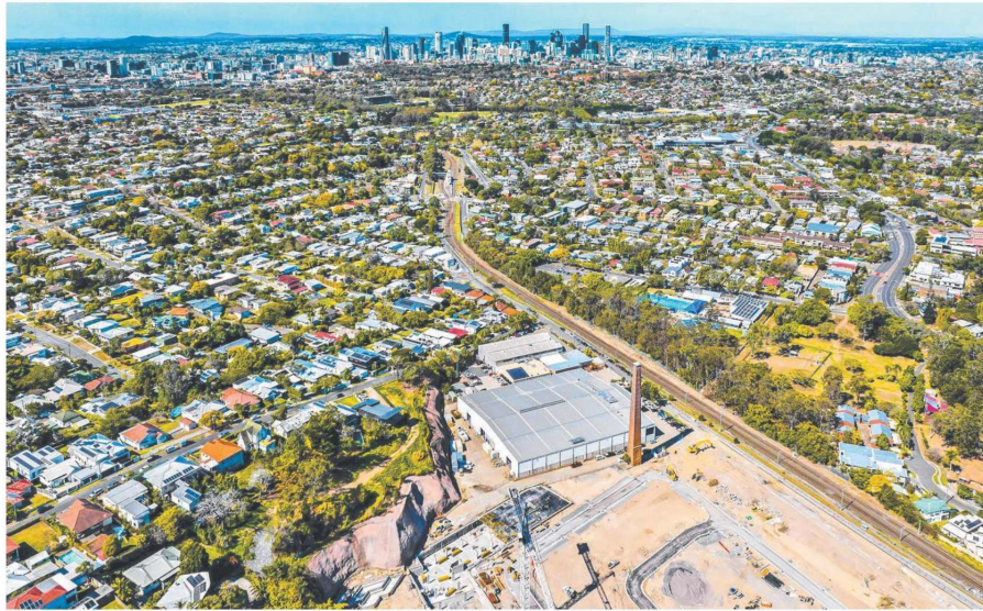
Centennial paid $13.7m for the 9089sq m site 95 Mina Pde, Alderley, that is leased by a Boeing Co subsidiary.
